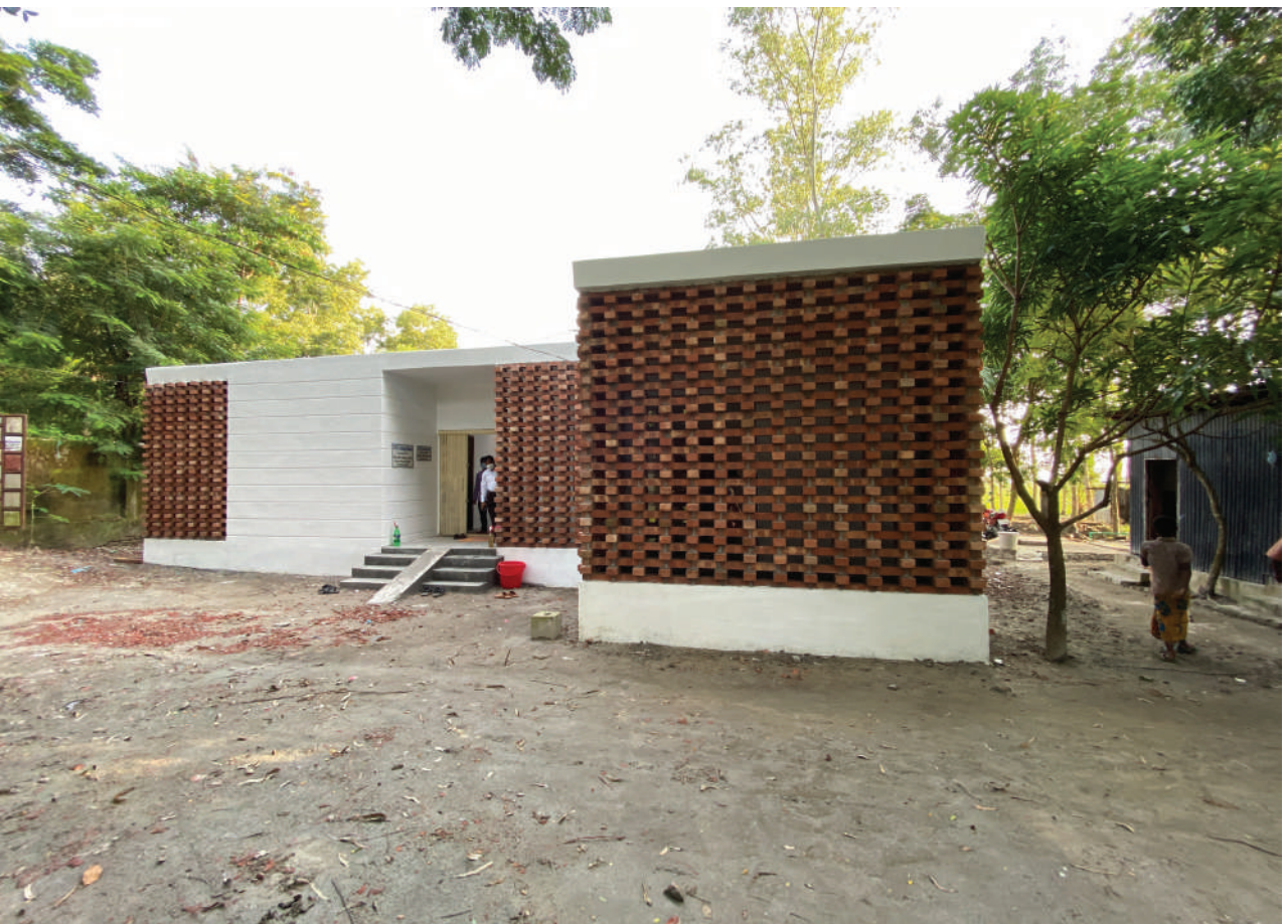
CODEC MF Office, Chotobogi, Potuakhali
