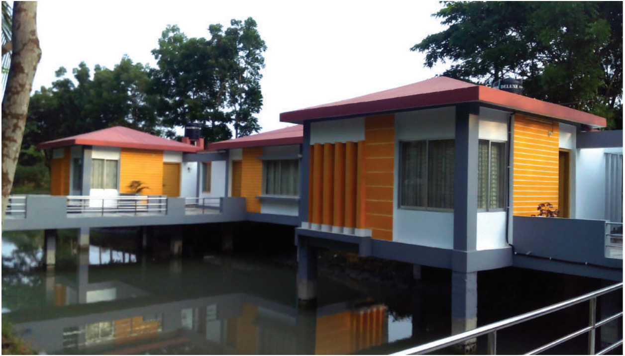
Cottages at CODEC Training Center, Potuakhali
