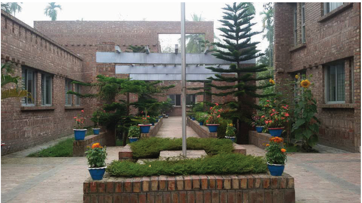
CODEC Training Center, Bagerhat
